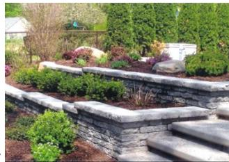
**Retaining wall** holds earth behind it or supports another structure or takes on additional load. The finished grade behind is typically at the height of the wall....
